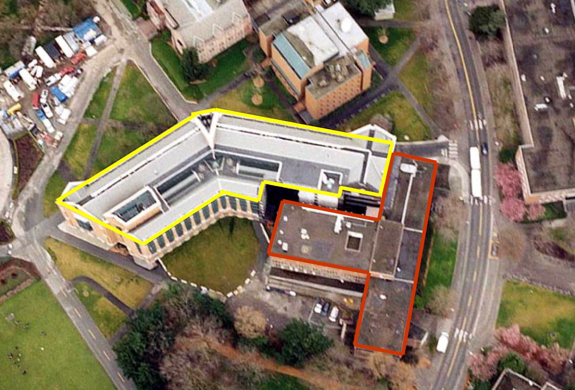
New and old EE buildings, 1998
