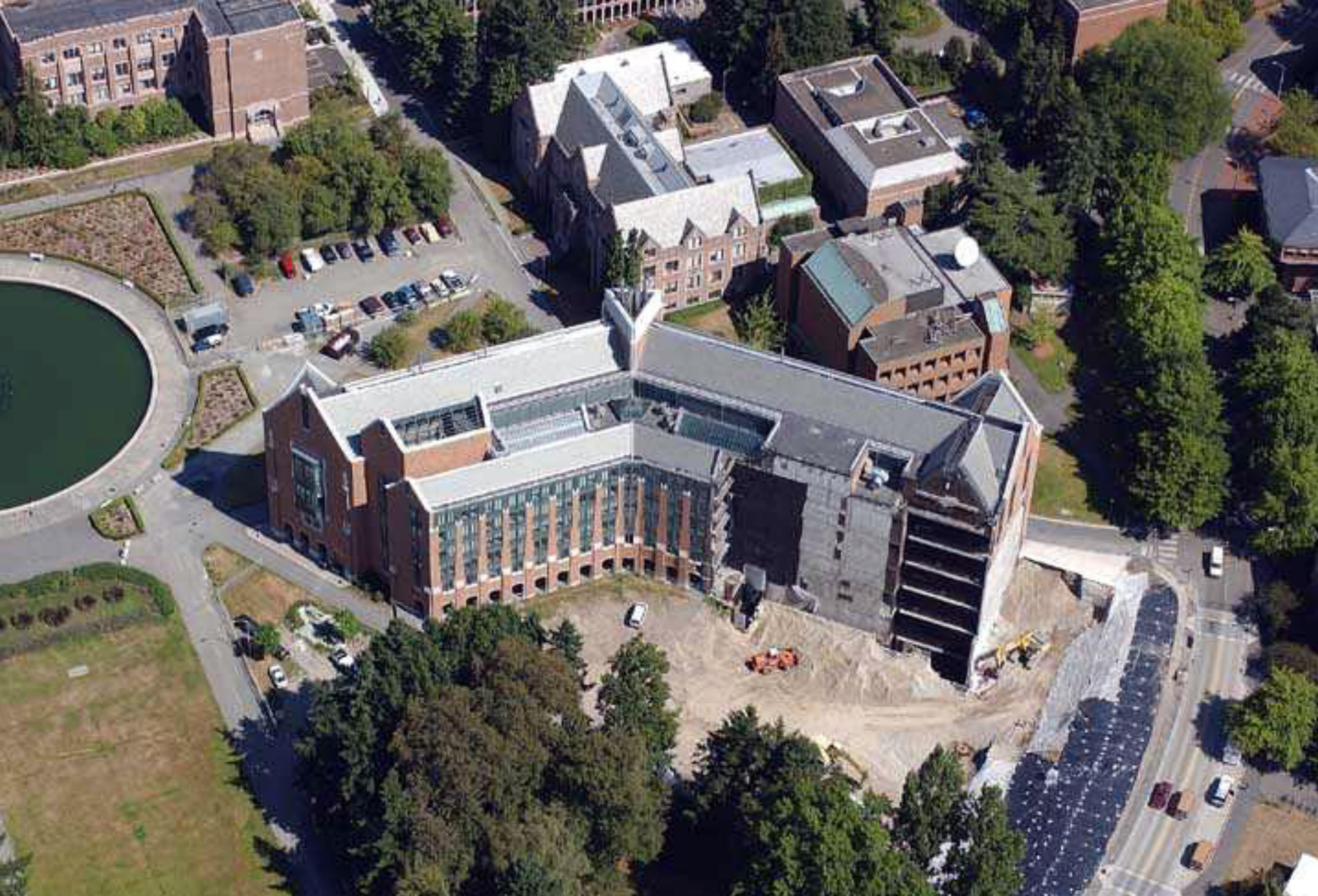
Demolition of old EE building, 2001
